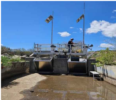
Baca-Picketwire – New automated headgate installation – April 2024
