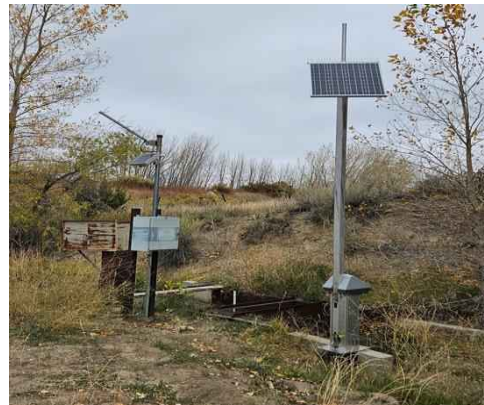
John Flood Ditch New automated headgate installation – October 2024
