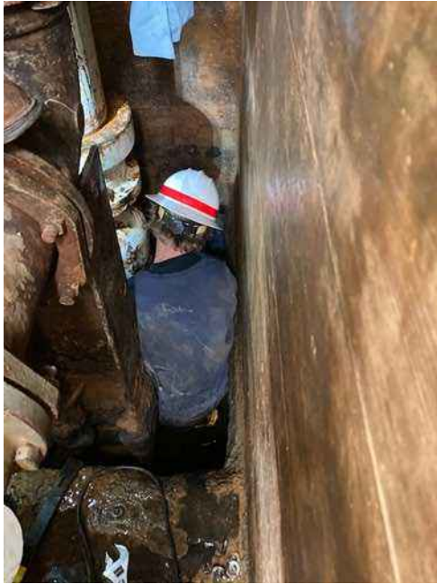
Figure 8: John Martin employee working to replace sump pump gasket.
