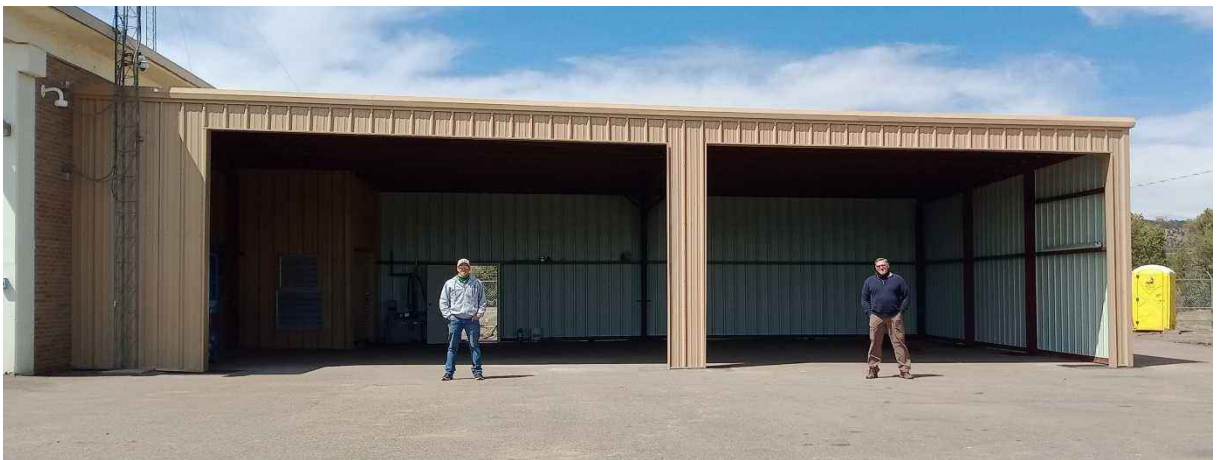
Figure 7: New heavy equipment shed and emergency generator storage at Trinidad Dam
